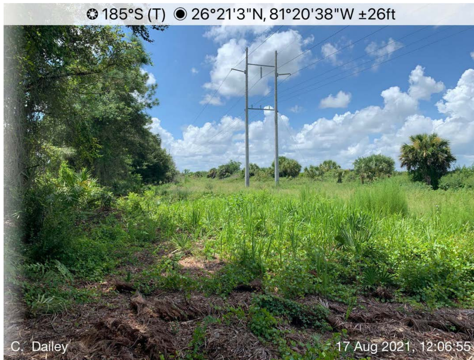
Photo 3: Electric Utility Corridor
